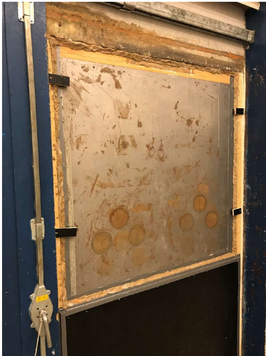
Figure 5: Prior to test measurement on the reference case “Mineral wool in slit and double-sided clay caulking” (see Appendix 5).
