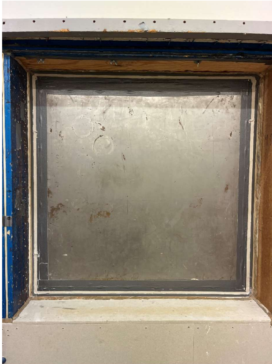
Figure 3: The fire stop mortar (white) at double-sided application from sending room
